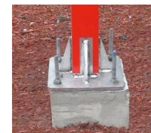
Clearance Structure Mounting
