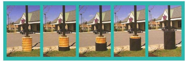
Concrete light pole bases will be covered with a 9.5'' tall ring set. A second ring set will extend the unit vertically to 19''. The third and fourth ring set will extend the unit vertically to 28.5'' and 38''. A two-piece cover will be installed upon the last ring set. This top section will have a cut out area at the light pole location that will be 1/8'' larger than the size of the light pole. A four-ring Poletector covers a standard 40'' base including the bolt cover.
