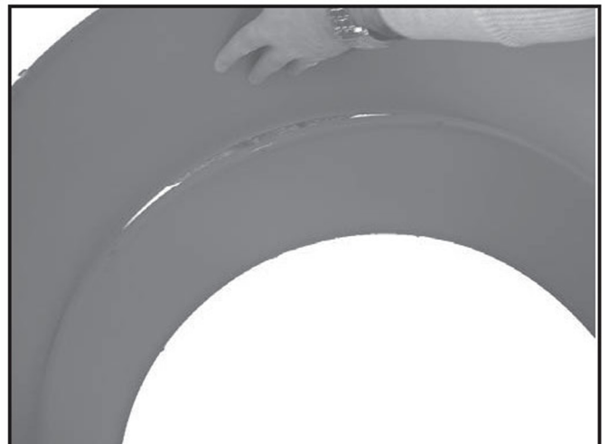
Work the horizontal seams together
