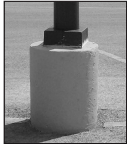
Level the ground around the base
