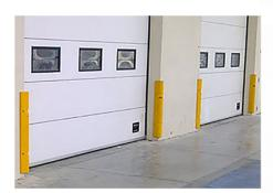
Anywhere a wall corner is exposed to vehicle traffic, Corner Sentry provides an energy absorbing barrier that protects the underlying building, the vehicle and the vehicle operator.
