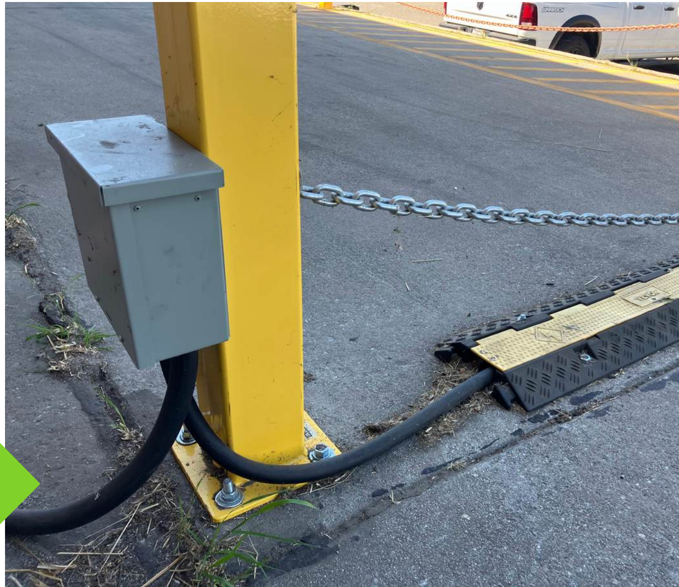
Raceway for AC connection
