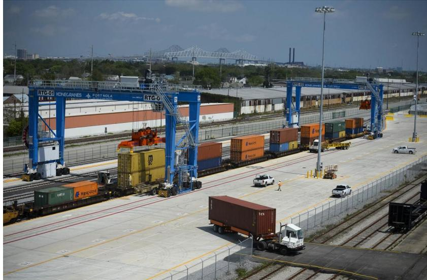
The \$24 million project involved the reconfiguration and relocation of an existing 12-acre rail yard into an efficient rail intermodal terminal container transfer facility at the Napoleon Avenue Container Terminal and 4 acres of paving improvements at an adjacent marine facility, the Louisiana Avenue Terminal.
