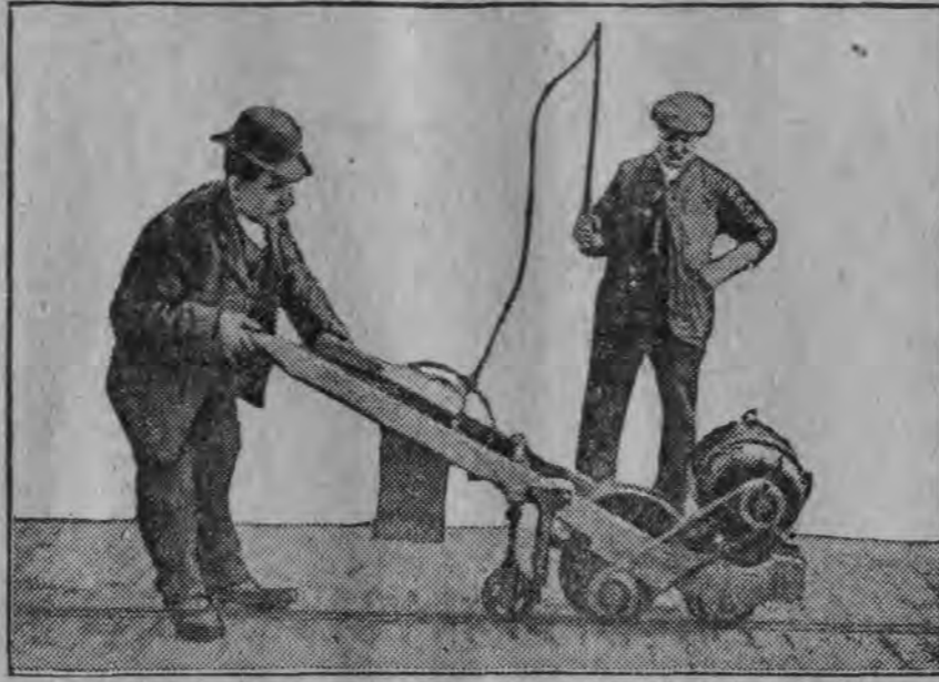
Grinding a Defective Rail-Joint With a Hand-Controlled Machine.
