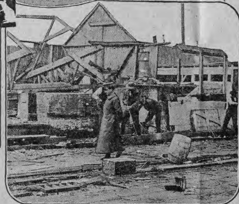
DEMOLISHING A "RAT ROOKERY"
