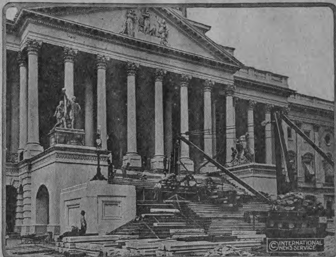
Workmen putting in new marble steps at the capitol at Washington to replace the old sandstone steps which time and the weather had rendered unsightly.
