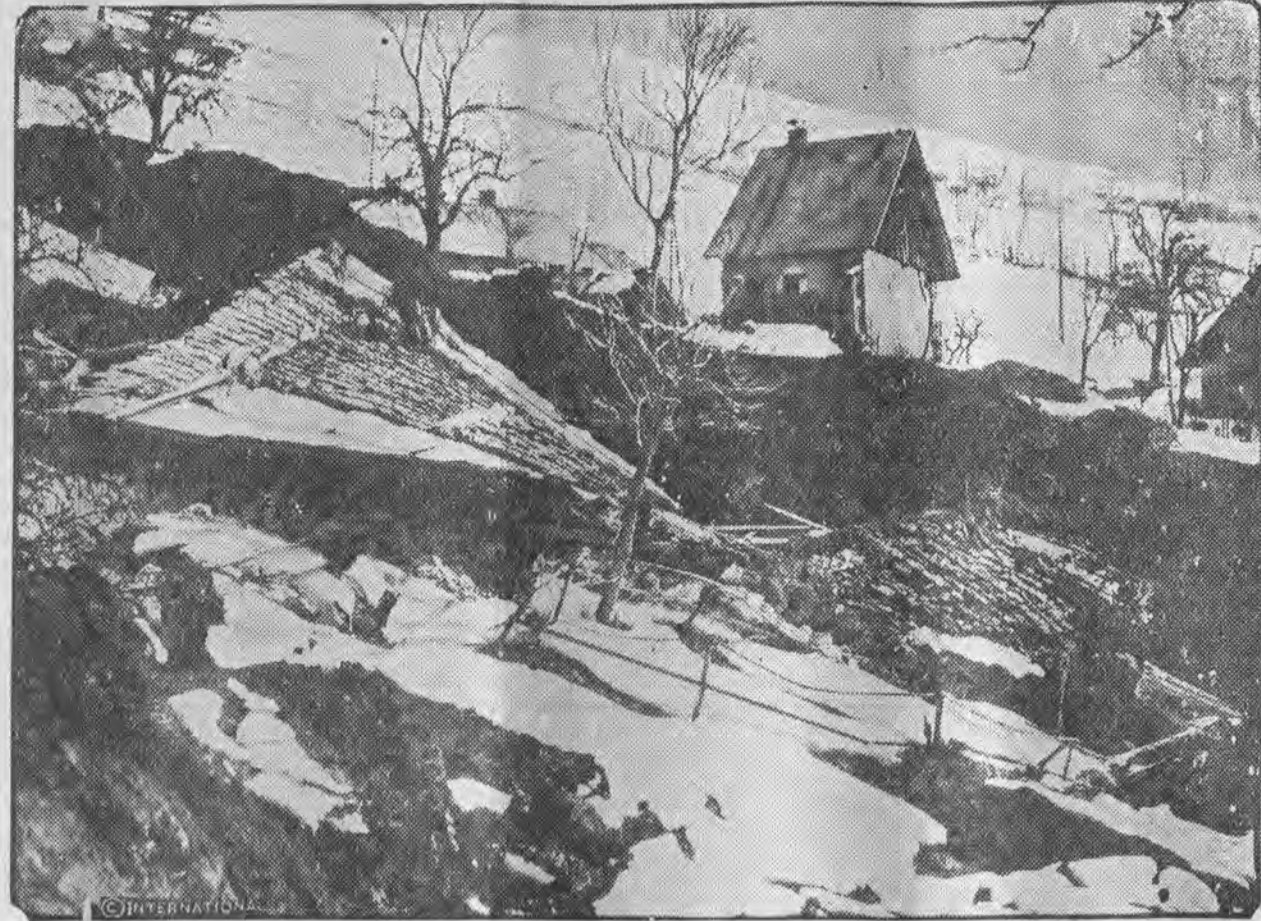
Silently, but remorselessly, a mountain of mud swept down the mountainside in the Bauges district of France recently, and destroyed two villages with its tremendous, irresistible force. The house in the foreground was carried away, with only the roof of the structure remaining. The onslaught of mud traveled at a rate of 200 feet an hour and caused terrified villagers to flee from their homes.
