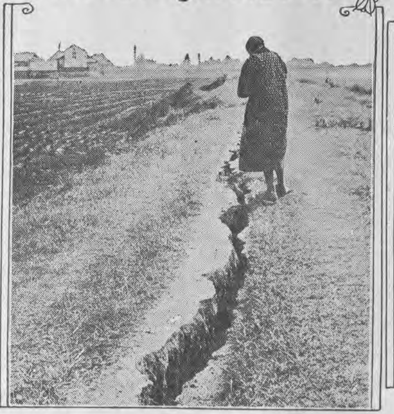
Crack in Filled Ground Caused by Earthquake in Japan.
