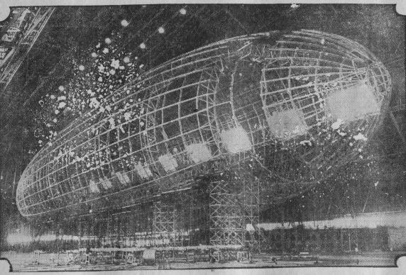
The world's largest dirigible, the Akron, being constructed for the navy at Akron, is rapidly nearing completion. Photo shows the metal skeleton of the huge ship.
