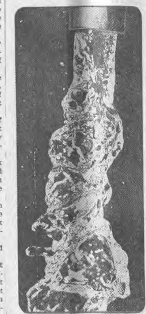
Water from the faucet stopped to pose for its portrait when this unusual photograph was made at an exposure of 1-50,000 of a second. The constantly changing pattern of flowing water, which ordinarily appears to the eye as a blurred vision, is now revealed in strange forms not unlike feeble or molten glass. The photograph was made by means of a new electrical circuit developed at the Massachusetts Institute of Technology by Prof. Harold L. Edgerton and Kenneth J. Gernsmauser.
