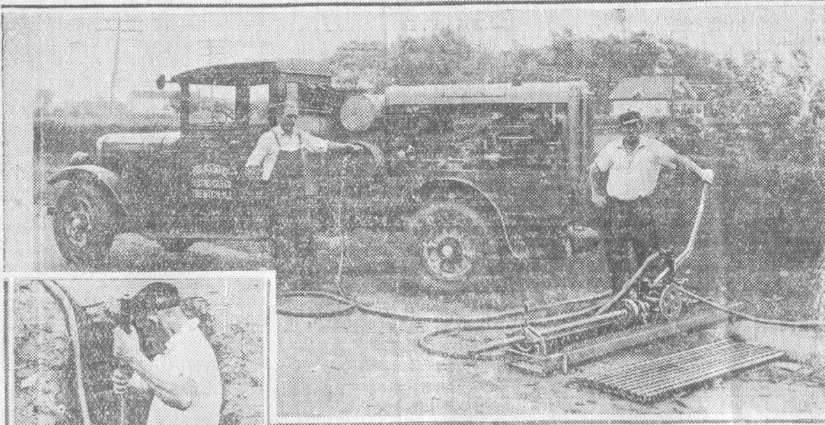
Above—Hydrauger with air compressor. Left—The machine in action.
