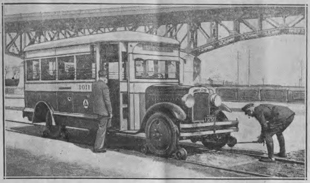
BUS equipped with an ingenious | device enabling it to run on steel tracks as well as on highways has been successfully tested by Public Service and the company contemplates putting It into operation on the "Fast Line" tracks between Trenton and Elizabeth. No specific date has been set, however. This is believed to be one of the first motor buses to be adapted for regular operation both on highways and on steel ralls.
