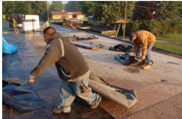
EPDM is removed from a ballasted system
