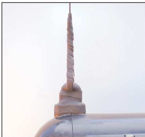
Properly installed probe using the direct connect method after application of rubberized electrical tape. Note that the tape is started at the plastic boss and wrapped upward.
