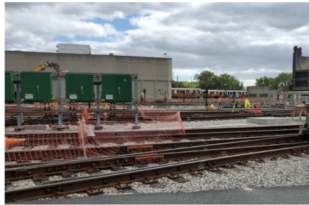
Crews work in Wellington Yard (September 2022)
