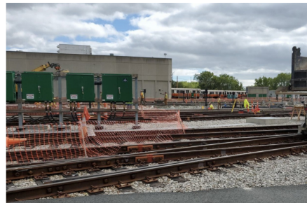
Crews work in Wellington Yard (September 2022)
