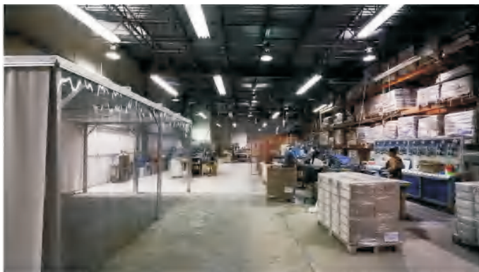
BEFORE: Production Area - 14 460W Metal Halide High Bays and 14 120W T12 8' Shop Lights cluttering up the space. = 8,120 Total Watts and very poor, uneven lighting.
