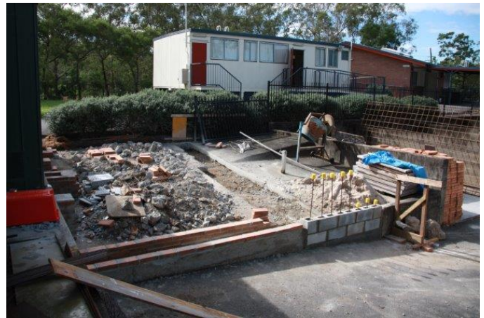
Work is in progress to add storage facilities behind the shed in to provide more space for workshop activities.
