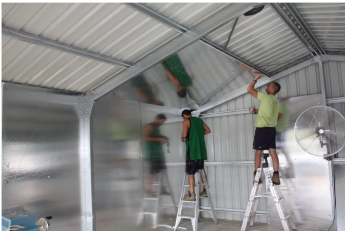
Installing the insulation was the first big job.
