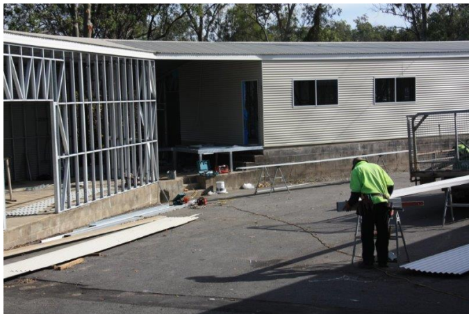
Construction of the Home Assist facilities behind the Shed are well advanced.
