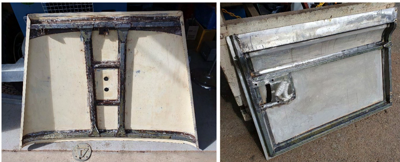
Underside of the bonnet and inside of the door showing the steel frame supporting the aluminium skin
