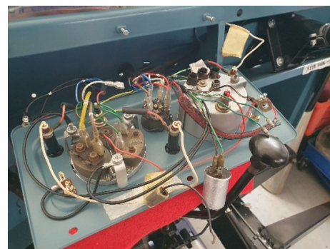
Rewiring in progress
