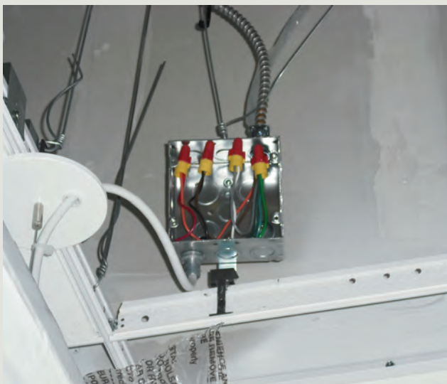
Light fixtures installed through a more effective process
