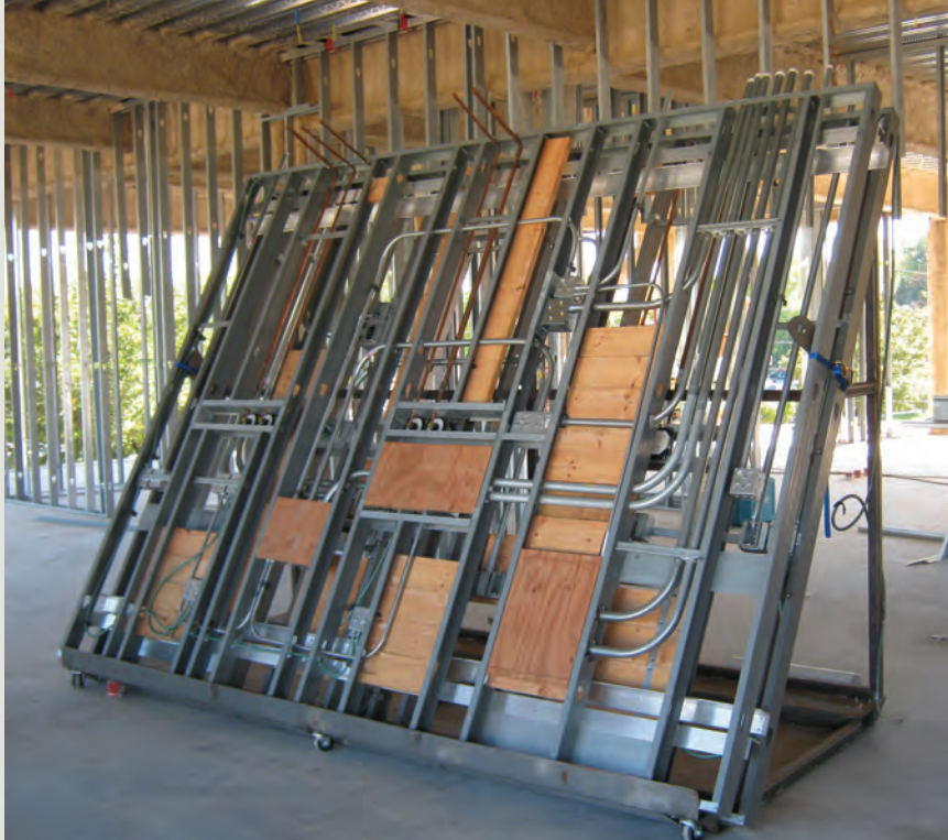
Headwall on the specially designed cart, prepped for installation
