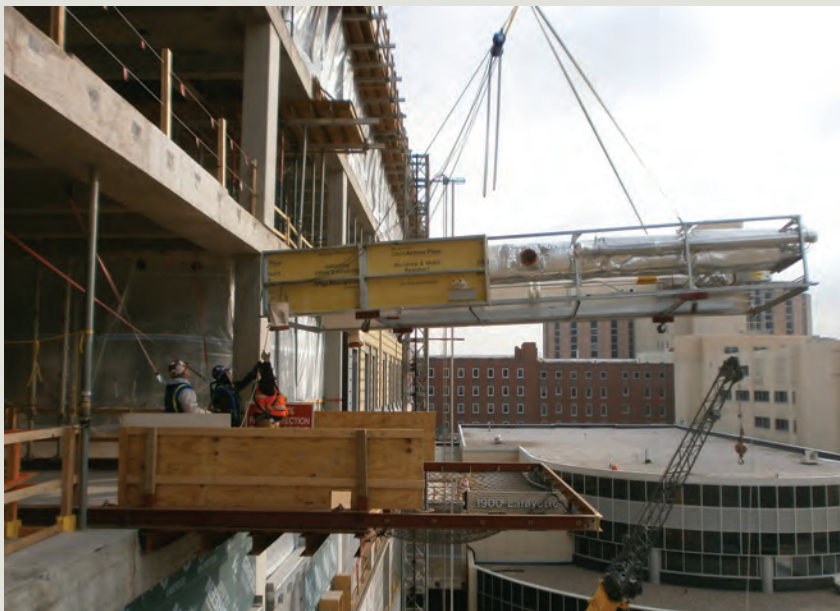
Crews built 166 multi-trade racks that are built in a warehouse and trucked to the site for just-in-time delivery.
