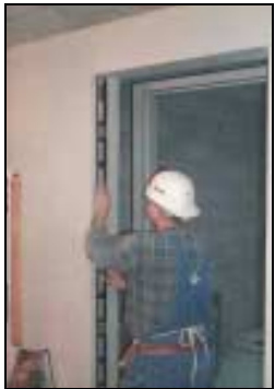
Figure 4: Drawing a Plumb Line
