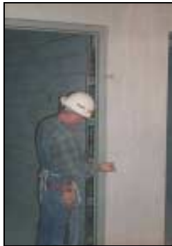
Figure 5: Inserting Wooden Shims
