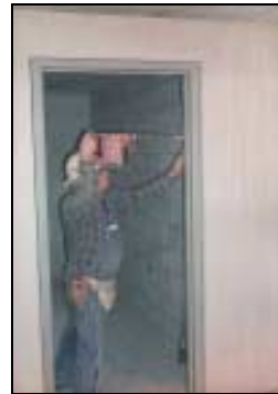
Figure 6: Drilling for Anchor Bolts
