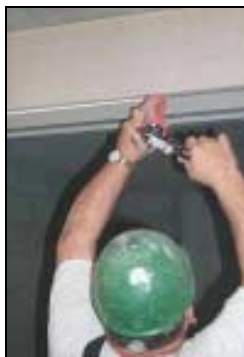
Figure 8: Caulking along the Top
