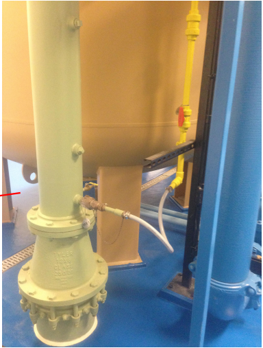
PRE-FILTRATION CHLORINE INJECTION POINT
