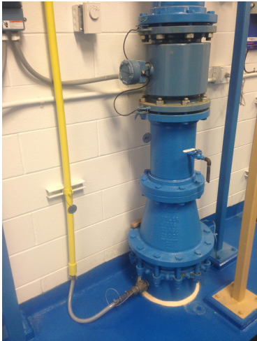
POST-FILTRATION CHLORINE INJECTION POINT
