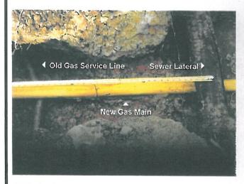
A blocked sewer line may be the result of another utility line (gas, electric, or communications) having been accidently bored through the sewer line.
