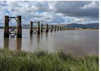
career, Mallard was sold on the 10th of February 1920 to the Alloa Ship Breaking Company for breaking. As a result of these incidents, three stone piers were replaced by cast iron ones and additional cross-bracing was added to all piers. Repairs were carried out by Sir William Arrol and Company, the contractor who helped build the Forth Rail Bridge.
