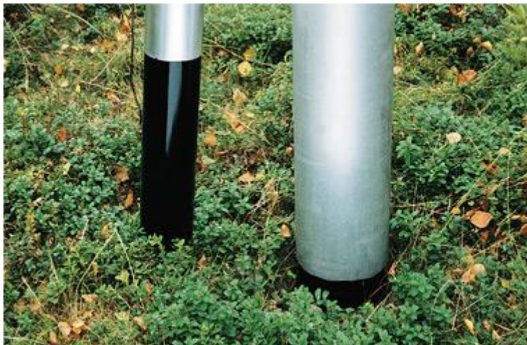
Bitumen coating prevents corrosion
