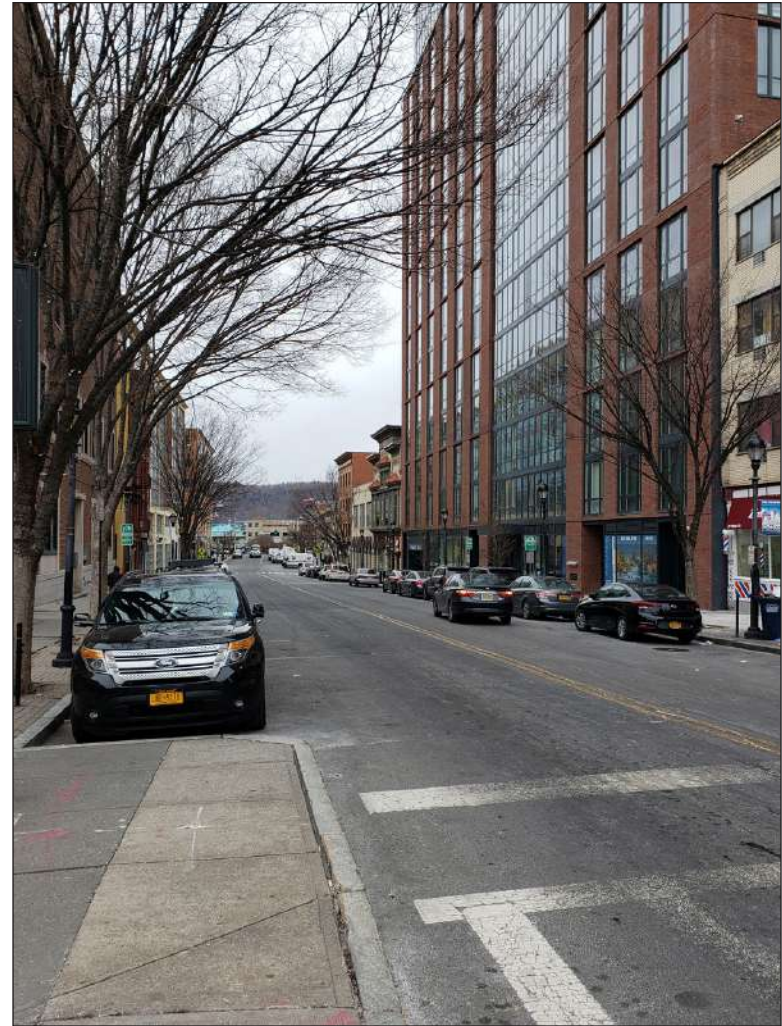
View west on Main Street 19
