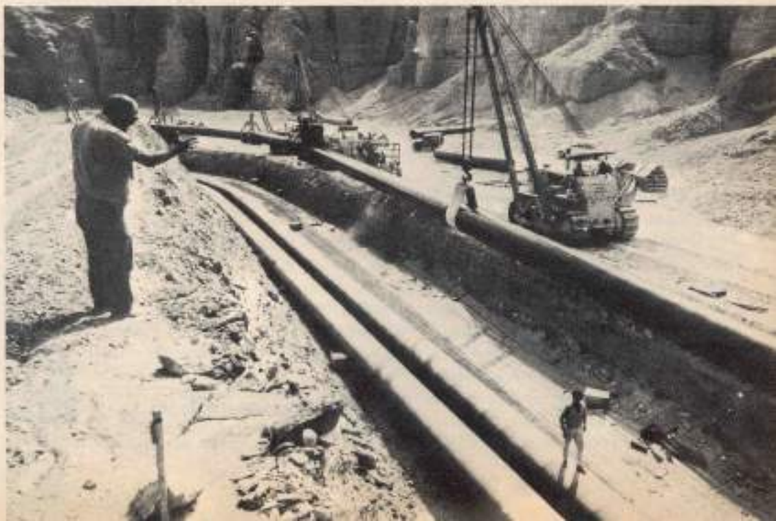
BY-PASSING THE SUEZ CANAL — the Israelis have completed a huge oil pipeline from the port of Eilat on the Gulf of Aqaba to Ashkelon on the Mediterranean. Tankers unload their cargo at Eilat. The oil is then carried by the pipeline to Ashkelon, where it is again loaded on ships and sent to Europe. The Israeli pipeline eliminates the long trip around the southern tip of Africa, as well as the now-impossible Suez Canal.
