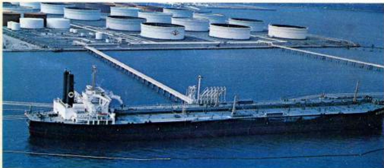
ONE OF THE WORLD'S LARGEST TANKERS , the 372,698 DWT Nisseki Maru , at Kiire Terminal. Located in Kogoshima Bay, Japan, the terminal is currently equipped with 12 oil storage tanks to hold petroleum shipped from Middle East.
