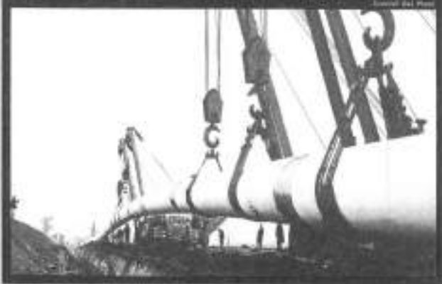
ACTIVE: BRITAIN'S first North Sea production platform "Giantstep 7" being towed down Solent Channel on its way to offshore orbit. BELOW: A section of 36" pipeline is hoisted into position for its lowered into trench.
