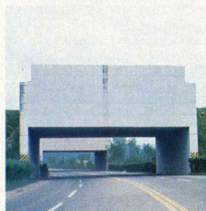
COLLAPSIBLE OVERPASS is designed to impede enemy wartime advance.
