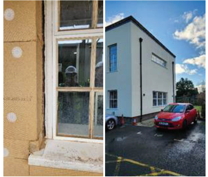
FIGURE 9 AND 10: EXTERNAL SOLID WALL INSULATION APPLIED TO THE SOUTH DOWNS CENTRE, MIDHURST 2023- 2024.
