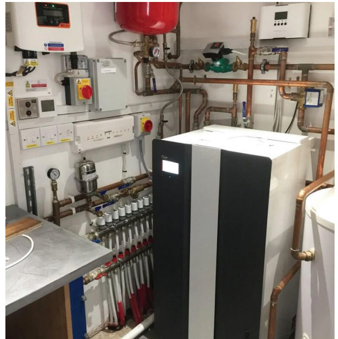
FIGURE 23: TYPICAL PLANT FOR DOMESTIC HEAT PUMP (WWW.SELF-BUILD.CO.UK)
