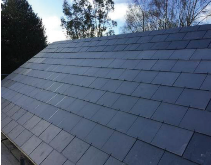
FIGURE 17: LOW VISUAL IMPACT PV TILES ON A SLATE ROOF
