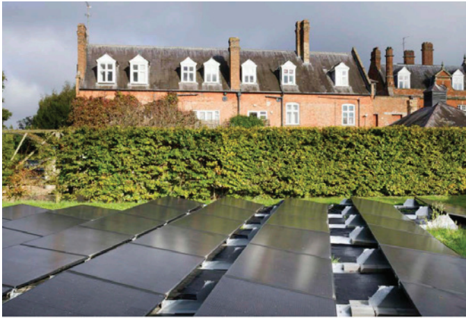
FIGURE 19: GROUND MOUNTED SOLAR PANELS IN A GARDEN (HE ADAPTING HISTORIC BUILDINGS FOR ENERGY & CARBON EFFICIENCY 2024)
