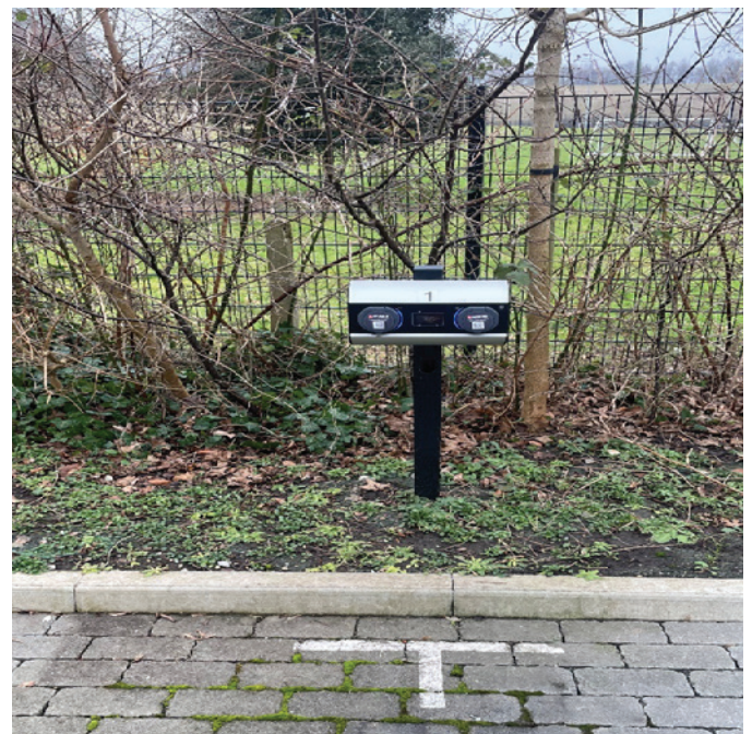
FIGURE 26: FREE STANDING DOUBLE CHARGE POINT IN RESIDENTIAL CAR PARK, MIDHURST
