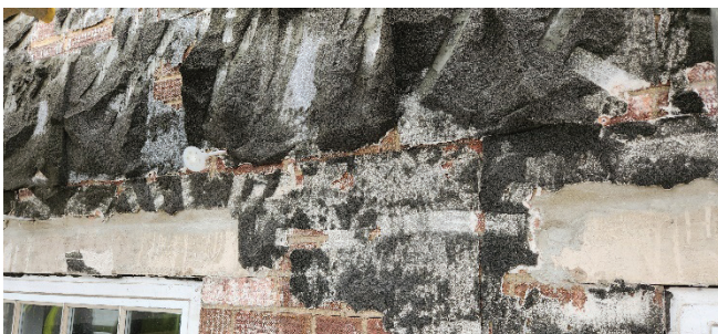
FIGURE 8: EXTERNAL SOLID WALL INSULATION APPLIED TO THE SOUTH DOWNS CENTRE, MIDHURST 2023- 2024. REMOVAL OF EXISTING RENDER ABOVE.
