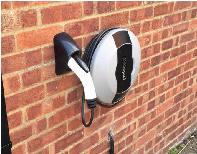
FIGURE 28: A WALL MOUNTED CHARGE POINT
