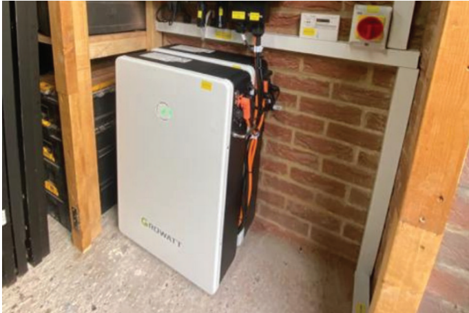
FIGURE 25: A TYPICAL DOMESTIC SCALE BATTERY STORAGE UNIT LINKED TO PV ON A ROOF (SOLARPANELINSTALLERS.UK)
