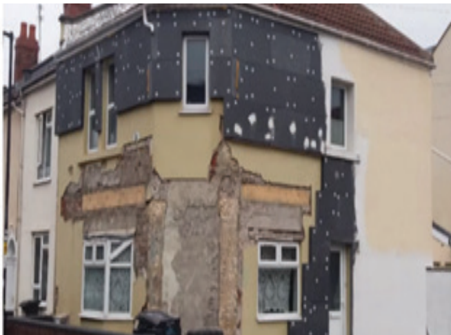
FIGURE 7: AN EXAMPLE WHERE THERE WAS A LACK OF UNDERSTANDING THAT THE BUILDING WAS A SHOP, WITH CORNER DOOR AND LARGER WINDOWS, WITH A MIXTURE OF FABRICS, CAUSING MORE ISSUES WHEN INSULATING. (HE)
