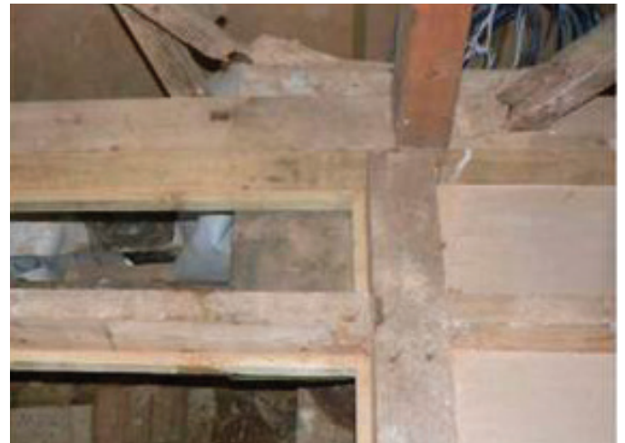
FIGURE 4: BATTENS ADDED AT THE SIDES OF THE JOISTS TO SUPPORT BOARDING & CARRY COMPRESSIBLE SHEEP'S WOOL INSULATION IN A SUSPENDED FLOOR
