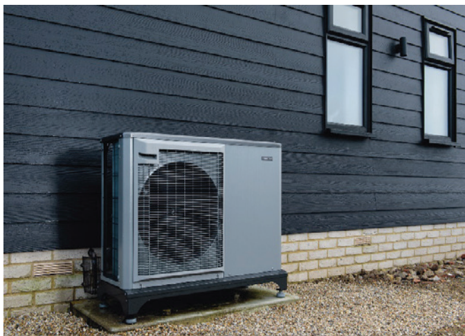
FIGURE 20: A TYPICAL DOMESTIC-SCALE AIR SOURCE HEAT PUMP (SELFBUILD.UK)
