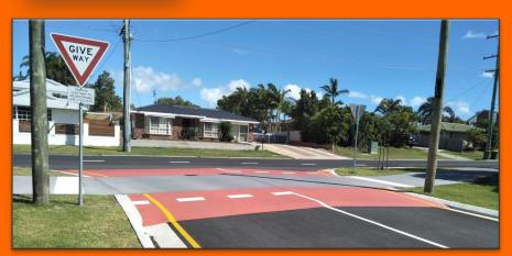
Where pathway users are given priority across a road using regulatory Give Way or Stop signs and line marking, it is referred to as a priority crossing. (Raised Priority Crossings for Pedestrian and Cycle Paths, TMR, 2019)
