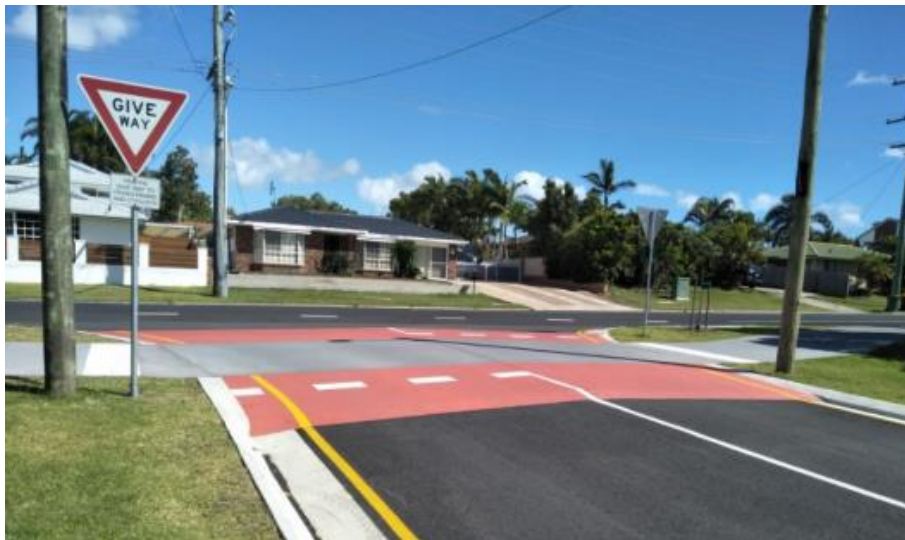
Figure 1: Raised Priority Crossing, Goonawarra Drive, Mooloolaba
