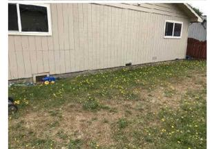
6. Marginal Swale: Flat or negative slope - Recommend improvements be made to the grade, swale slope and depth to improve water control
