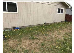
5. Swale: Flat or negative slope - Recommend improvements be made to the grade, swale slope and depth to improve water control
