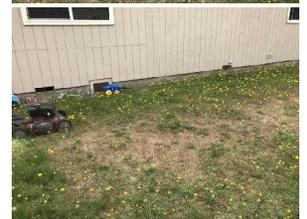
6. Exterior Surface Drain: Surface drain - Evidence of poor drainage at the down spouts. the down spouts are discharging next the foundation which can lead to foundation settling issues along with introducing moisture into the crawl space. I recommend adding extensions to help divert water away from the foundation.
