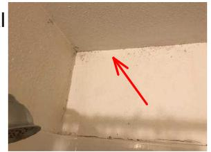
27. 1st floor main Bathroom Tub/Surround: Fiberglass tub and fiberglass surround - Replace caulking at the base of the tub is recommended.
