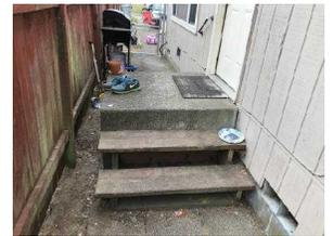
5. Marginal, Defective Grading: Flat - The Grading has a flat negative slope and water can pooling against the foundation. Noted along the back side of the house. Under heavy rain conditions water may accumulate around this area cause water to pool up against the foundation. Efforts should be made to improve grade and or add a French drain system to help divert water away from foundation
