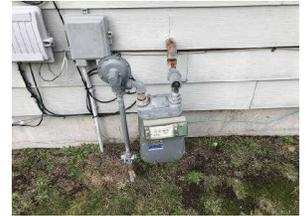
14. Acceptable, Marginal Main Gas Valve: Located at gas meter - I recommend a gas wrench be tethered to the meter so it is easy to turn off the gas in an emergency situation.
