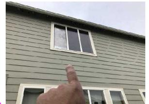
9. Marginal, Defective Window Screens: Vinyl mesh - **Noted some of the window screens were missing and I found others that were damaged or torn. Repairs and replacement recommended.**
