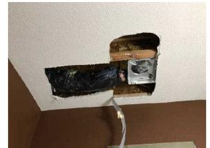
18. 1st floor main Half Bathroom HVAC Source: none - No heat source found in this bathroom?? Further evaluation from a heating contractor is recommended to ensure a heat source is present or installed in this bathroom.
