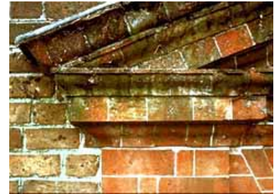
This 18th century pediment and surrounding wall exhibit distinctively different mortar joints. Photo: NPS files.
