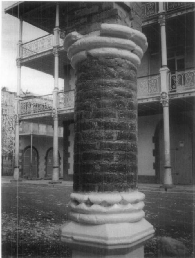
Figure 24. Although the application of a water-repellent coating was probably not needed on either of these buildings, the coating on the brick building (above), is not visible and has not changed the character of the brick. But the coating on the brick column (below), has a high gloss that is incompatible with the historic character of the masonry.
