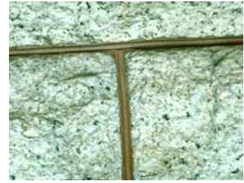
This late 19th century granite has recently been repointed with the joint profile and mortar color carefully matched to the original. Photo: NPS files.
