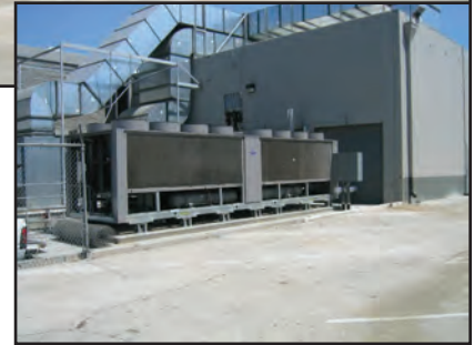
Chiller Barrier Wall System, Before (right), After (above)
