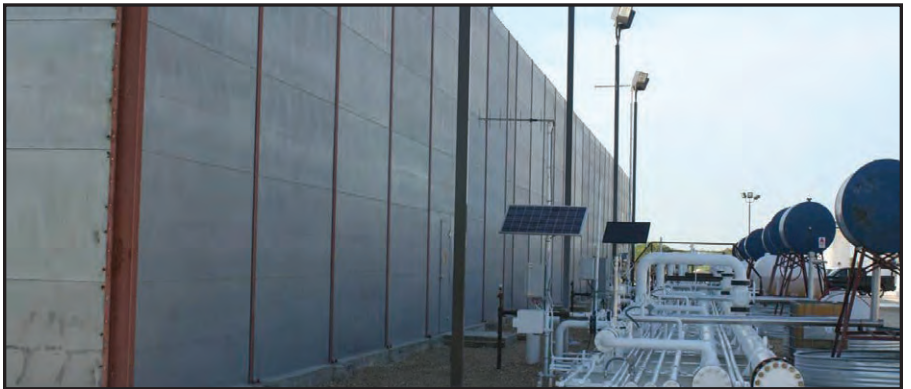
NOISEBLOCK™ Barrier Wall Midstream Compressor Station
