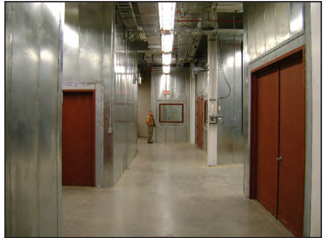
Control Room and Testing Enclosures
