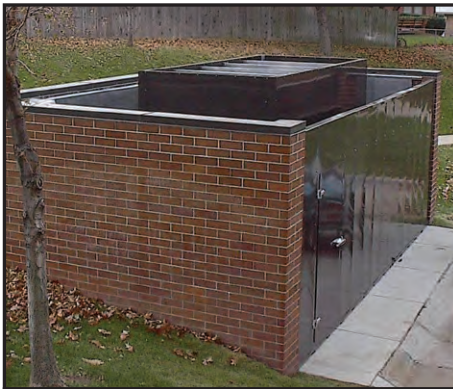
Chiller Barrier Wall
