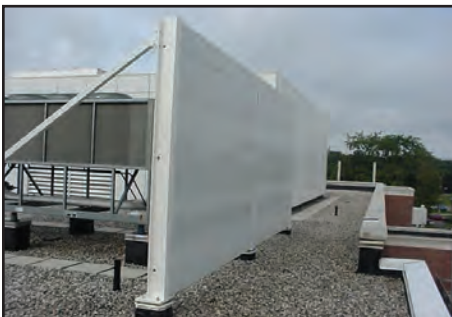
Roof Top Barrier Wall
