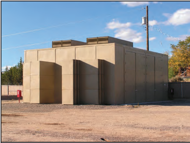
Dual Midstream Compressor Building
