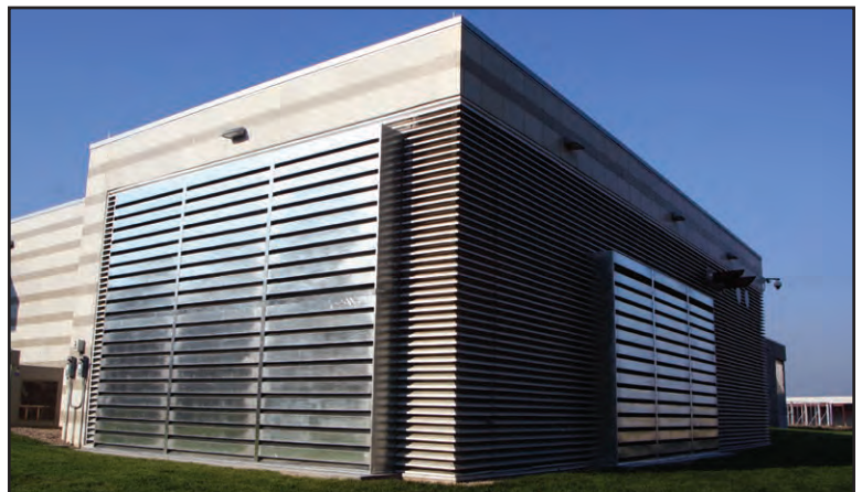
Data Center Backup Generators Room Louvers
