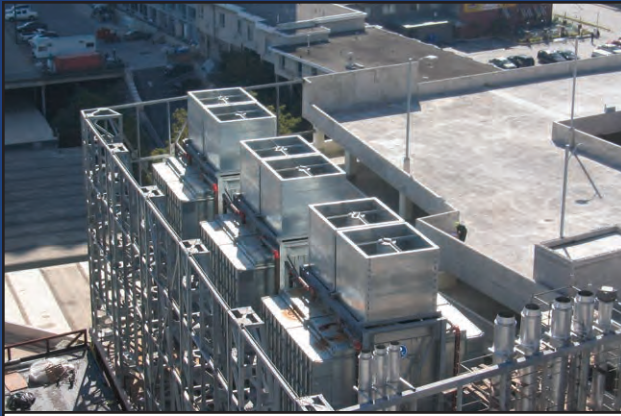
Custom Cooling Tower Ventilation Silencers
