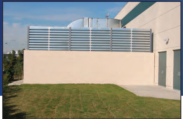
Equipment Yard Barrier Wall
