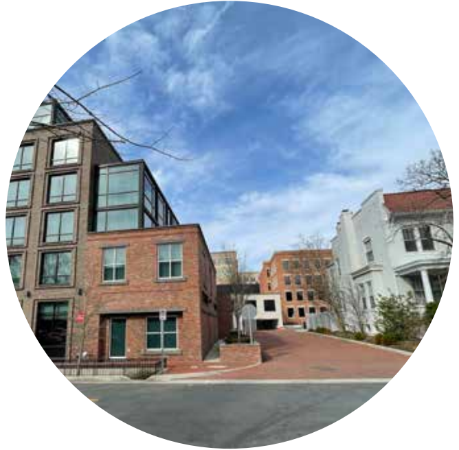
Alleyway and stepdowns in building height create a buffer and transition to existing single family homes
