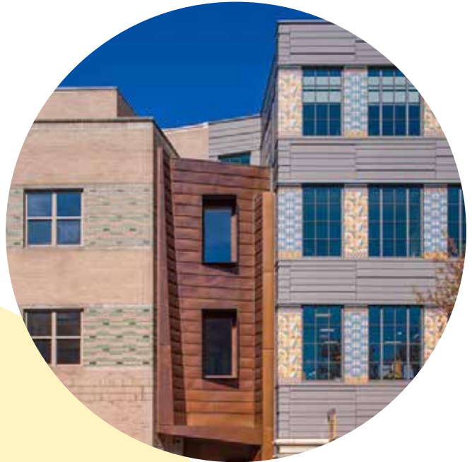
Use of masonry cladding and complementary materials can create variety in texture and building articulation
