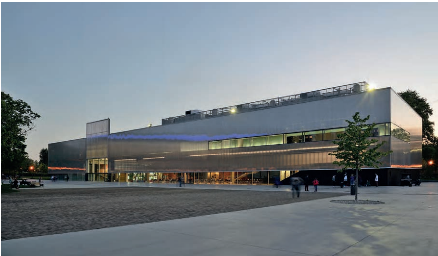
Exterior view of Garage building.
