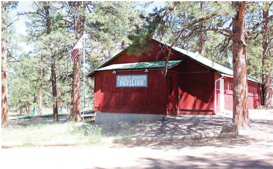
Casey Jones Pavilion in Casey Jones Park
