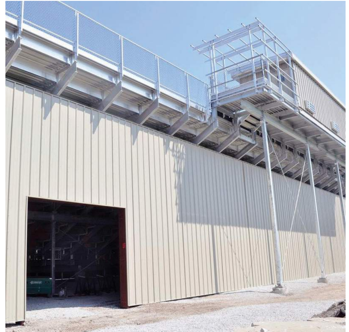
Opportunity for future maintenance facility under the Grandstands
