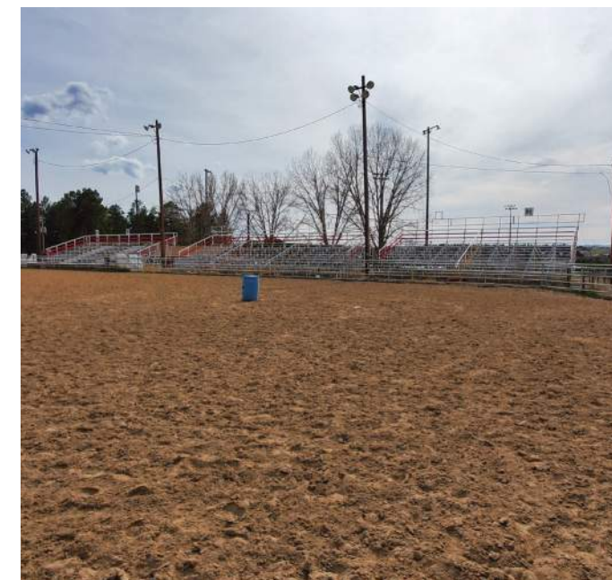
Existing rodeo arena
