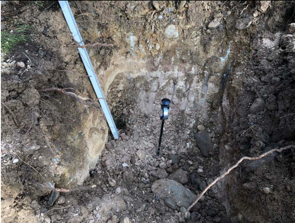
Description: TP-02 Cone Penetrometer pushed to 3 inches under a 320 psi loading.
