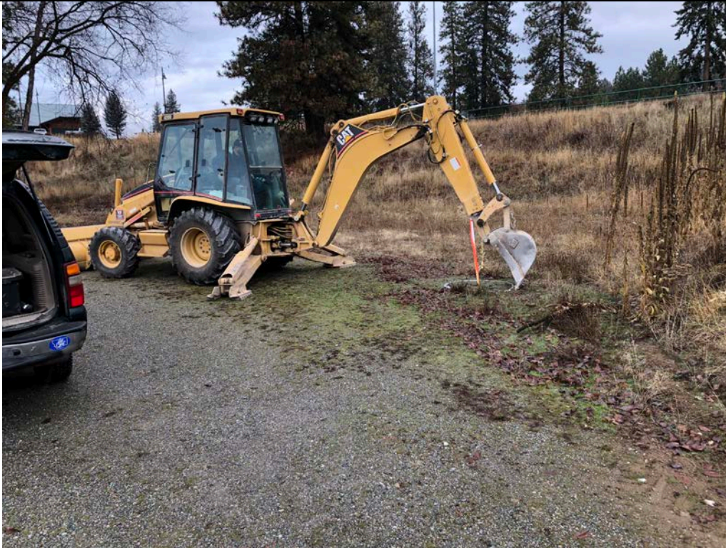
Description: TP-01 Location. View is to the north.
