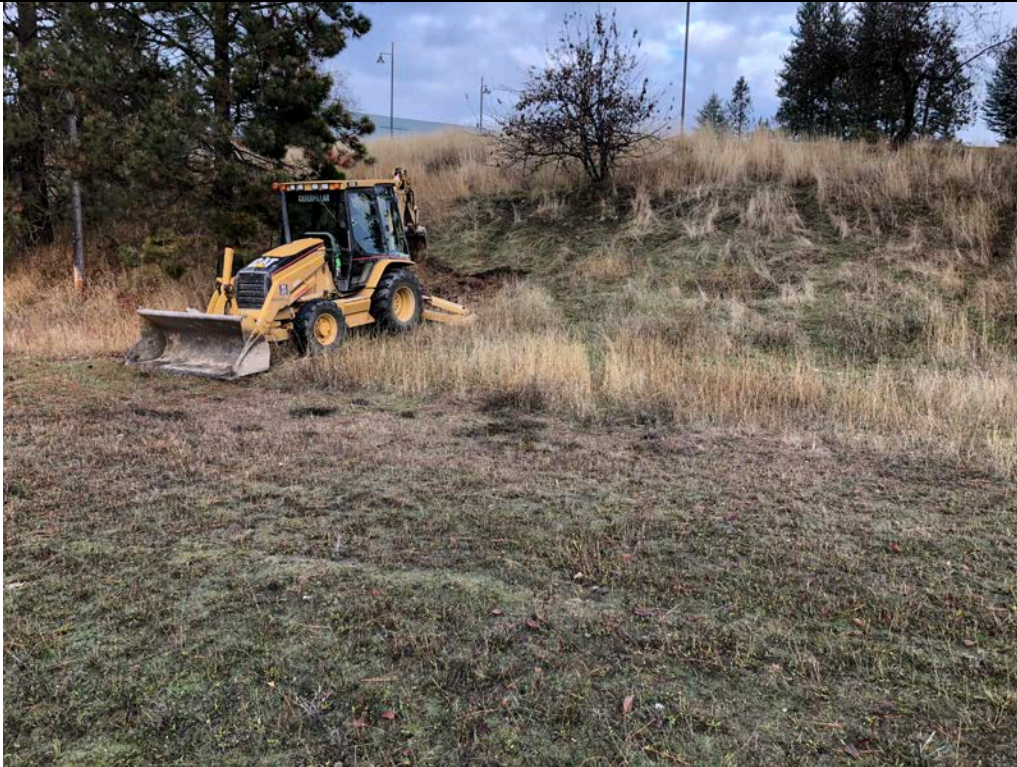
Description: TP-02 Location. View is to the north.
