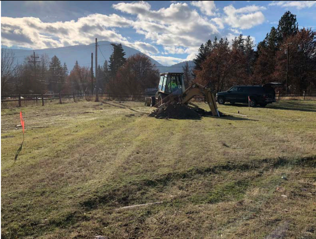
Description: TP-04 Location. View is to the south. Water utility trench depression is in the foreground.
