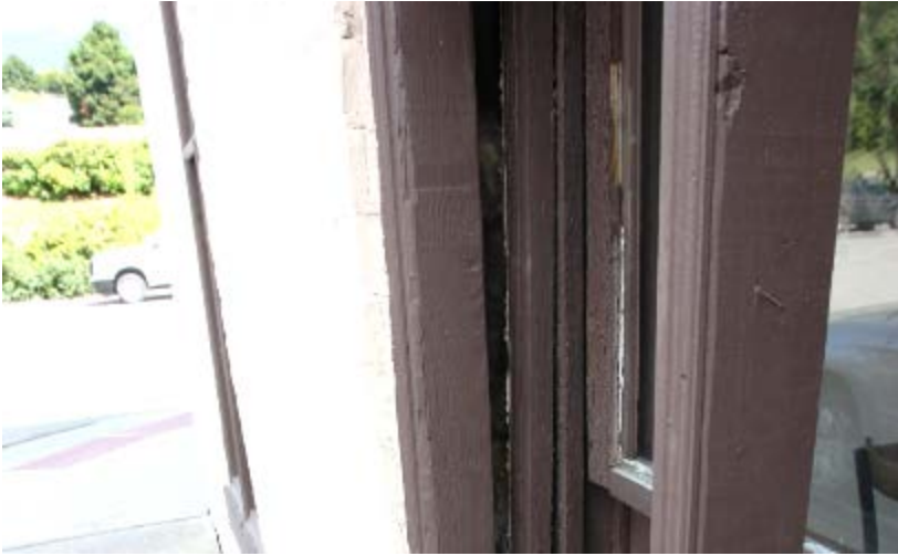
Figure 54: Black Bear Inn. The >2" gap between the brick veneer and the structure is probably indicated of insufficient masonry ties in the original construction.
