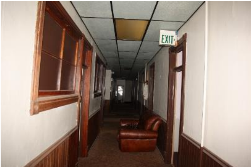
Figure30: Black Bear Inn. Second floor corridor with interior windows, transoms, and typical trim treatment. Photograph taken looking east.
