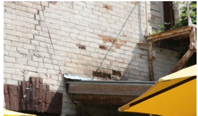
Figure 46: Black Bear Inn. Brick has spalled, mortar joints have cracked, and brick arches have expanded.
