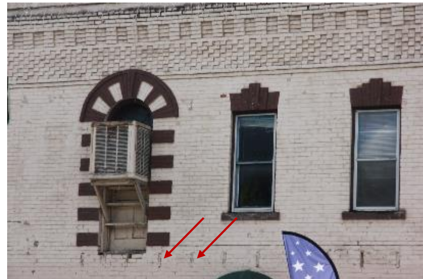
Figure 21: Black Bear Inn. The second floor opening to the original balcony (location evident by the joist pockets at arrow tips), with brick quoins accentuated by the alternating paint coloration.
