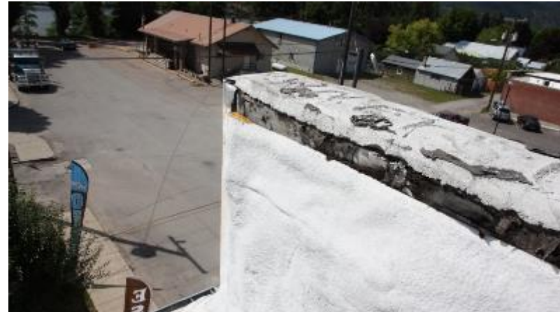
Figure 38: Black Bear Inn. Looking southwest at the exposed parapet wall's wooden sheathing.
