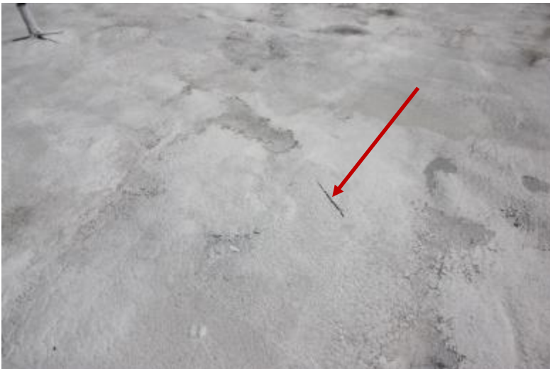
Figure 37: Black Bear Inn. The crack at the arrow tip is a typical condition of the roofing membrane.
