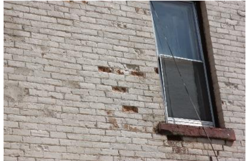
Figure 19: Black Bear Inn. The lug windowsills are of poured-in-place concrete.
