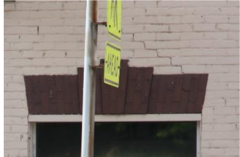
Figure 42: Black Bear Inn, north facade, showing a minor stepped crack above the jack arch of a first floor door.
