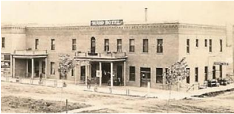
Figure 24: Black Bear Inn. Historic photograph depicting the five entry doors on the north façade, at left. Photograph courtesy of Daniel Moore.
