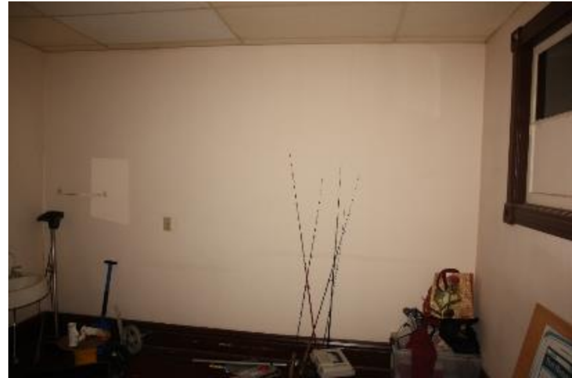
Figure 64: Black Bear Inn. The plaster walls are typically in good condition.
