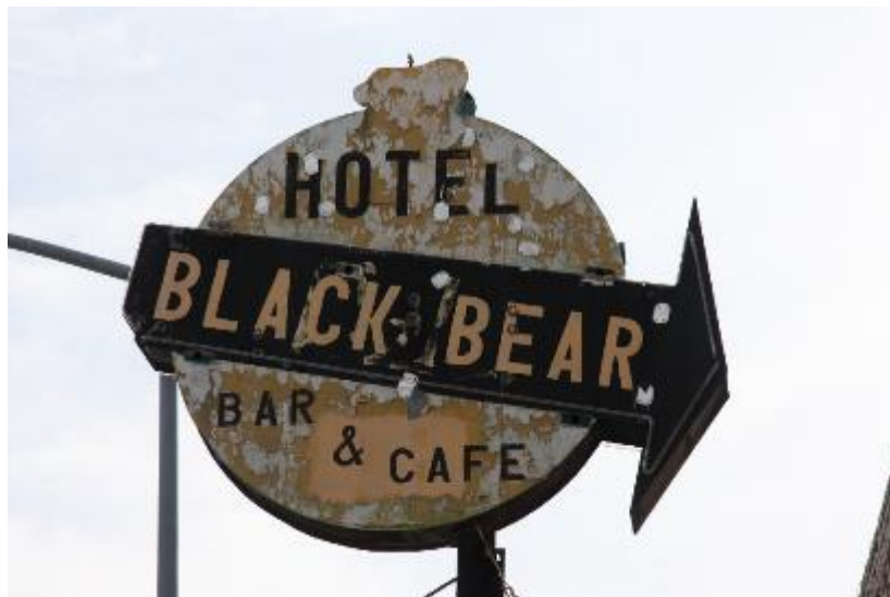
Figure 57: Black Bear Inn. The face of the historic Black Bear Hotel sign has numerous metal patches, presumably covering holes caused by rust.
