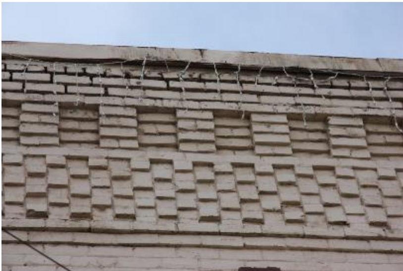
Figure 18: Black Bear Inn. The multi-course cornice, with corbeling and seed patterned brick, is the piece de resistance of the building.
