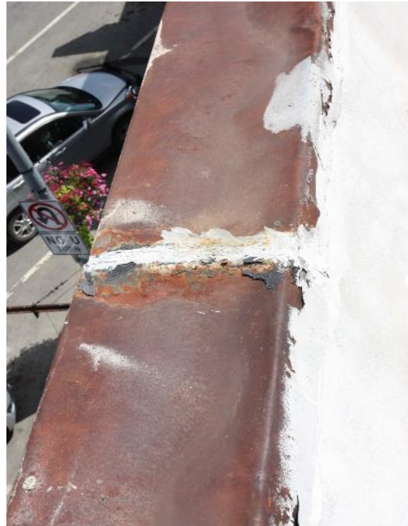
Figure 37: Black Bear Inn. Looking down at the rusted sheet metal coping of the front parapet. The sealant covering the joints has dried and cracked.
