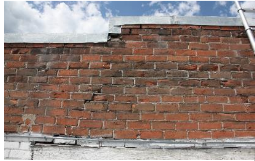
Figure 48: Black Bear Inn, east facade, where mortar is deteriorated at top 2-3 courses of brick.
