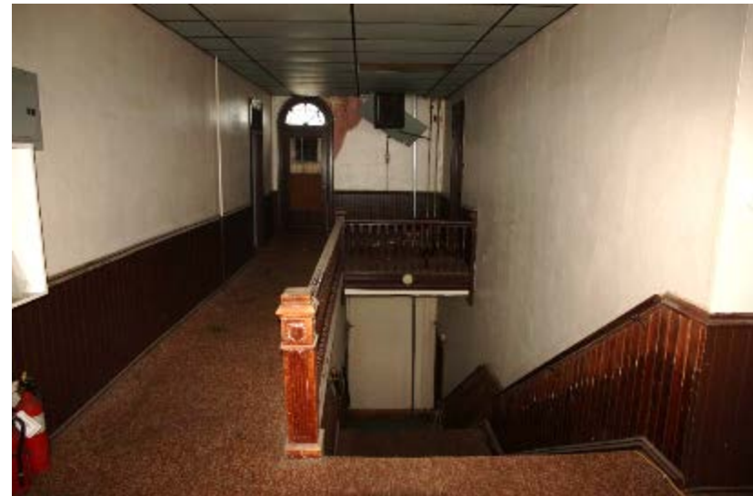
Figure 31: Black Bear Inn. The main interior stairway, looking down north to the first floor. The balcony door is at the landing by the far wall.
