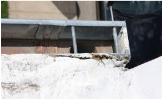
Figure39: Black Bear Inn. Looking down at the west end of the gutter. The bottom surface is rusting. The gutter is fastened to the wood fascia with a spike and ferrule system.
