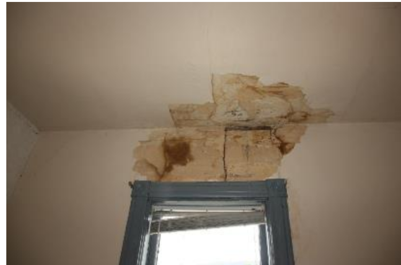
Figure 65: Black Bear Inn. Some of the exterior wall plaster has cracked and delaminated from water penetration.
