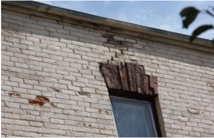
Figure 47: Black Bear Inn. Open mortar joints and spalled brick are the result of moisture penetration into the brick veneer.
