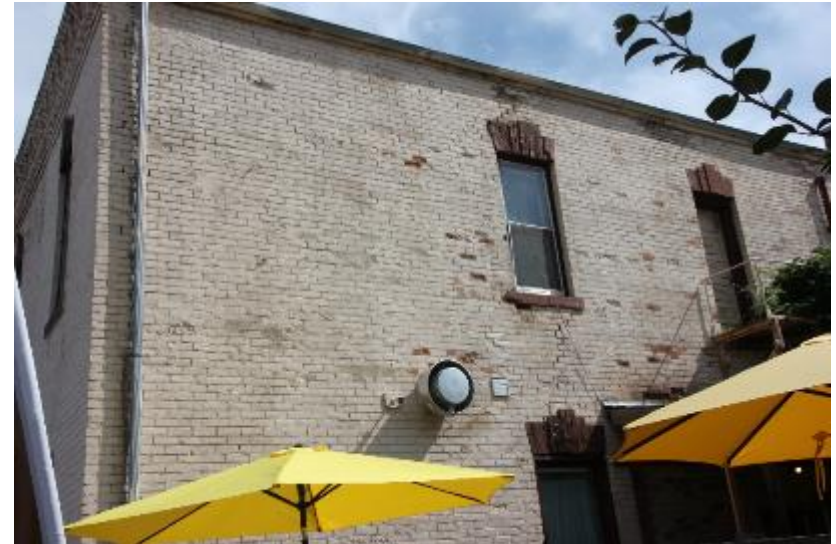
Figure 45: Black Bear Inn. The condition of the west portion of the south facade is representative of the façade. Water penetration has caused isolated brick to spall, mortar joints to erode (see cracking at arrow tip).
