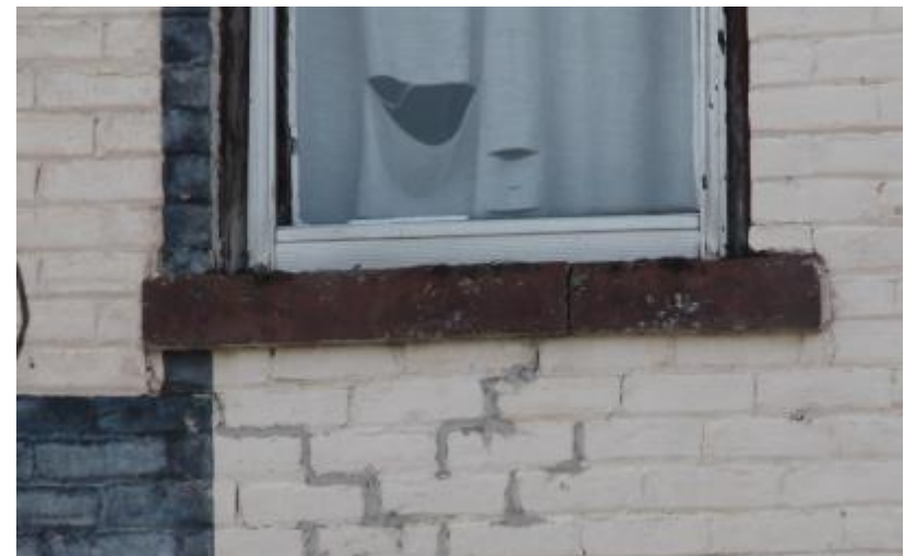
Figure 43: Black Bear Inn. The concrete sill of this second floor west facade window is cracked above the stepped crack in the brick below.
