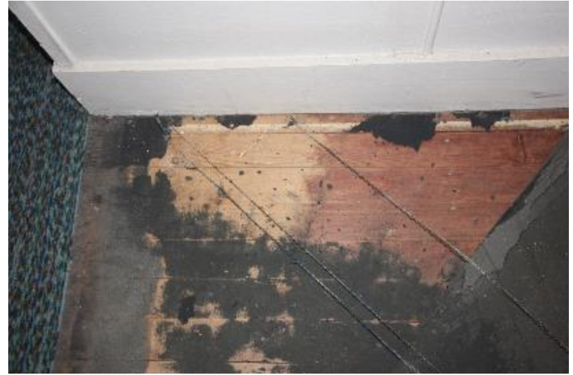
Figure 70: Black Bear Inn. Original wood flooring visible where the carpet has been pulled up in Room 11.
