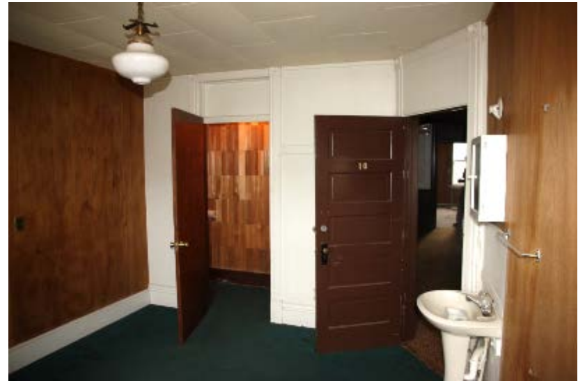
Figure33: Black Bear Inn. Typical second floor room with original paneled doors and transoms.
