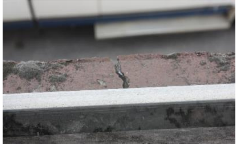
Figure 60: Black Bear Inn. Crack in exterior concrete windowsill at northwest window in Room 11.
