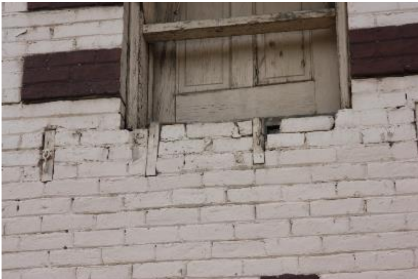
Figure44: Black Bear Inn. The door threshold at the second floor, north facade, does not appear to cover the brick veneer sufficiently.
