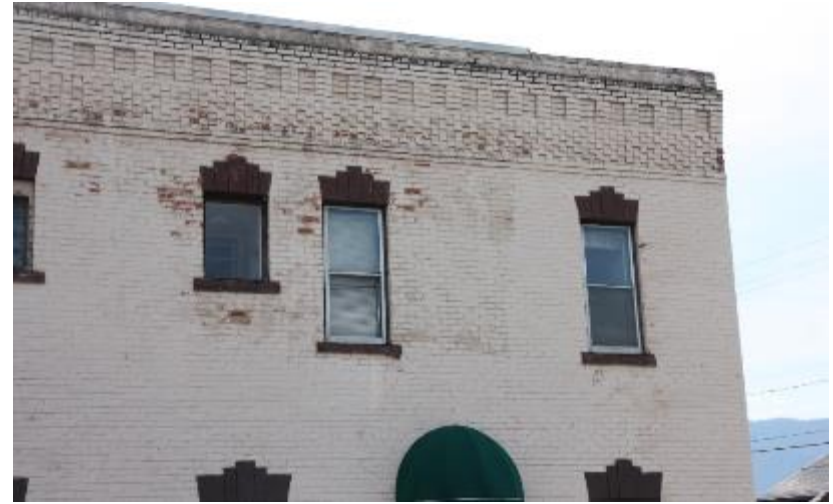
Figure 51: Black Bear Inn. Moisture has caused the top parging to crack and the paint to peel from the brick. Some of the brick have spalled.
