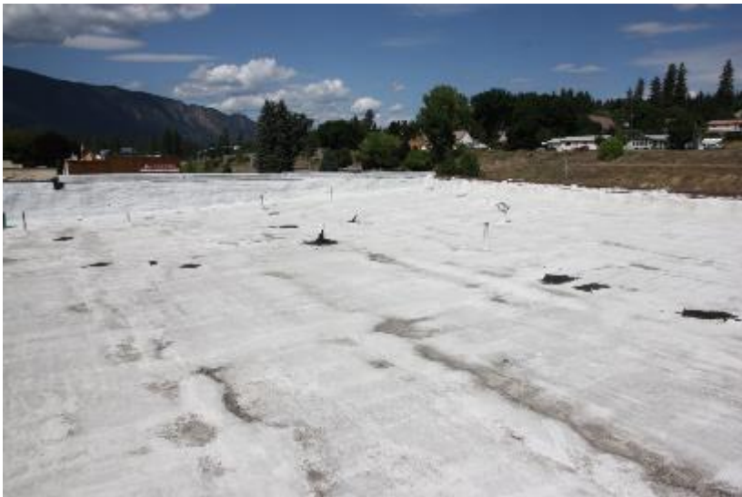
Figure 36: Black Bear Inn. Looking to the northwest across the slightly-sloped membrane roof.
