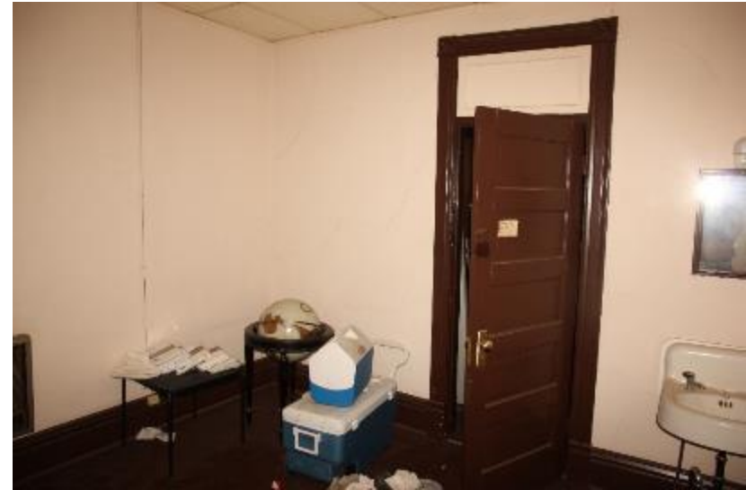
Figure 66: Black Bear Inn. Typical five panel door and painted transom.
