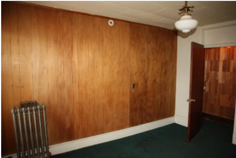
Figure 63: Black Bear Inn. Wood veneer paneling in second floor Room 10.
