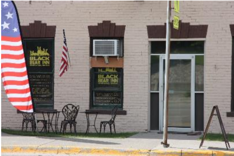
Figure26: Black Bear Inn. Westernmost first floor aluminum entry with sidelights and transom, within the original masonry opening.
