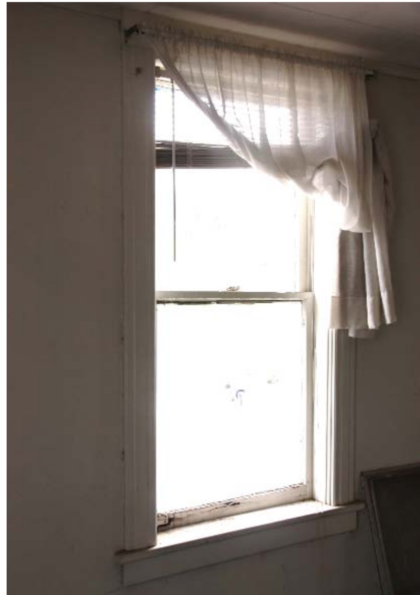
Figure 58: Black Bear Inn. The northwest window in Room 11 is representative of the typical window in the building. Room 11 is at the northwest corner of the 2 nd floor.
