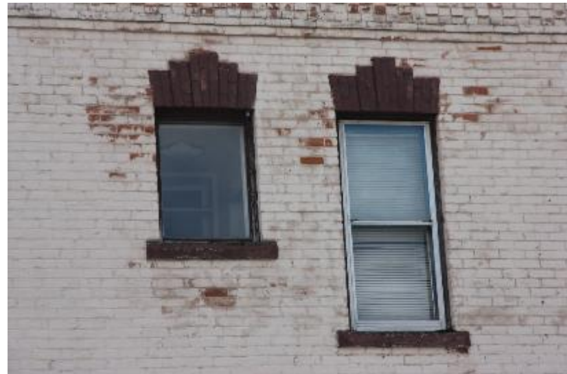
Figure27: Black Bear Inn. Typical double-hung window at right and shortened window at left, at second floor of west façade.
