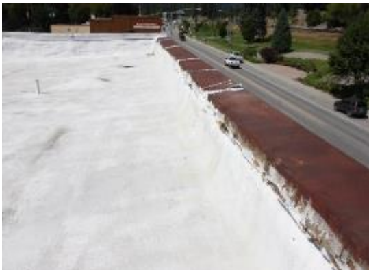
Figure40: Black Bear Inn. Looking west along the back face of the front parapet wall.
