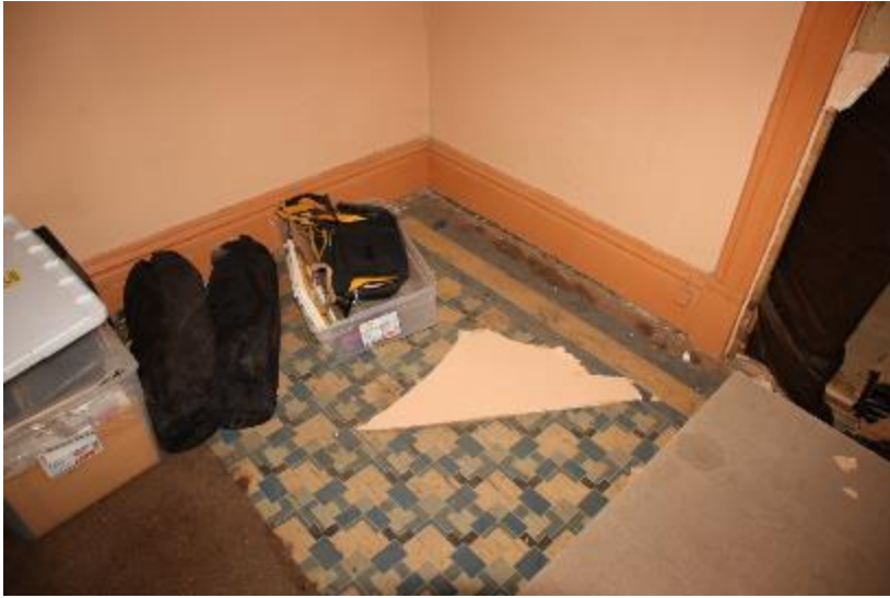
Figure 69: Black Bear Inn. Some rooms have sheet linoleum flooring underneath the carpeting.
