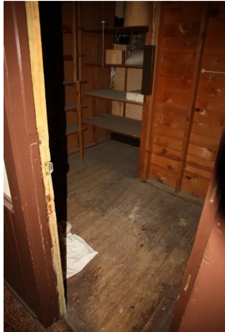
Figure 68: Black Bear Inn. The wood tongue-and-groove flooring in the second floor closet is indicative of the flooring throughout the second floor.
