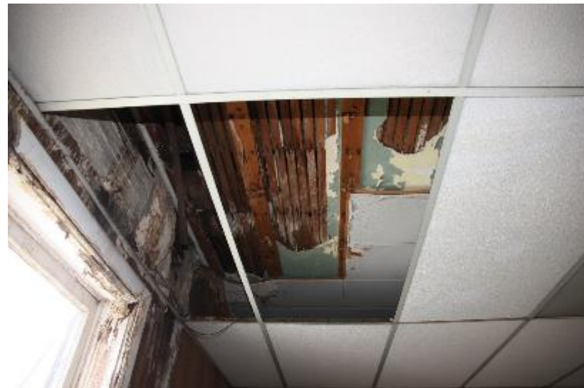
Figure 62: Black Bear Inn. Original plaster ceiling exposed above the fiberboard ceiling and suspended ceiling below.
