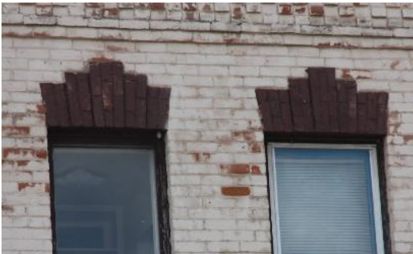
Figure 20: Black Bear Inn. Typical window head treatment of keystone brick.
