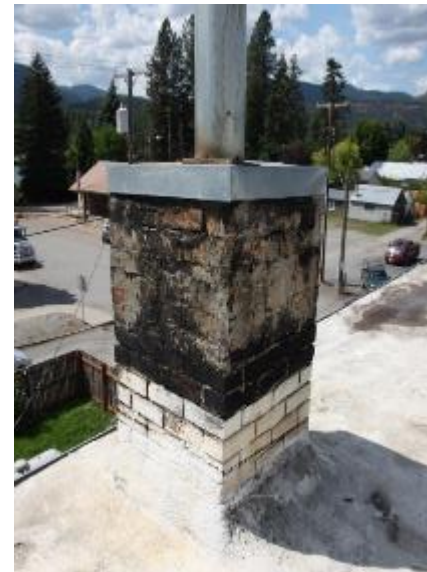
Figure 41: Black Bear Inn. The chimney is not properly flashed and the mortar joints have eroded.
