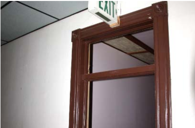
Figure32: Black Bear Inn. Typical corridor transom at second floor corridor.
