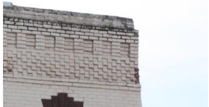
Figure 52: Black Bear Inn. Close-up of cracked and delaminated parging at west parapet.
