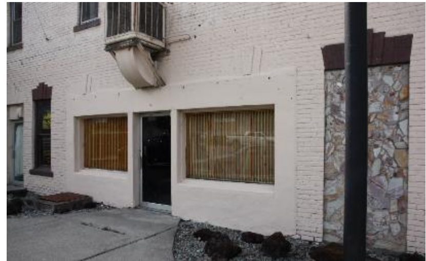
Figure 25: The first floor opening into the erstwhile dining room was updated with concrete c.1938. The center entry - to the right - has been infilled with stone.
