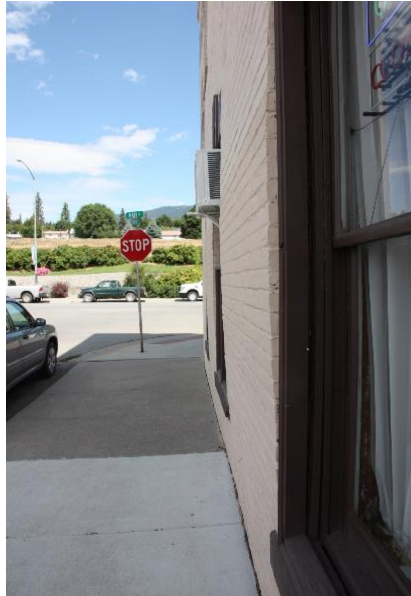
Figure 53: Black Bear Inn. Typical bowing of brick veneer at first floor of west elevation. Photograph taken looking north.
