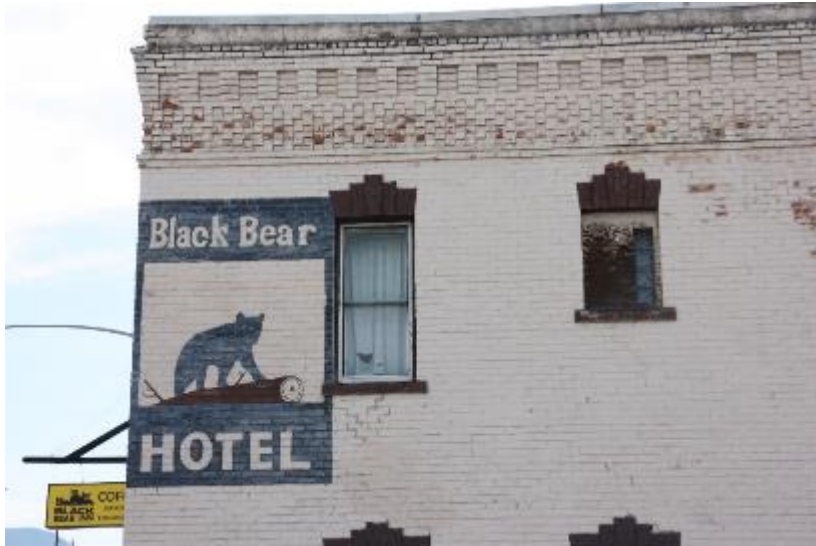
Figure 50: Black Bear Inn. Cornice of west facade. The upper courses of brick and mortar have eroded and loosened from water penetration at the coping.
