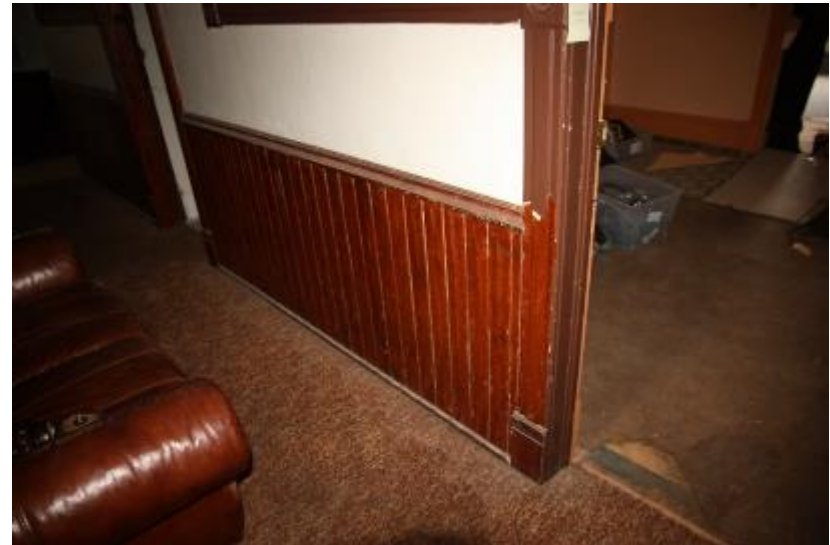
Figure34: Black Bear Inn. Original beadboard wainscoting on the second floor.
