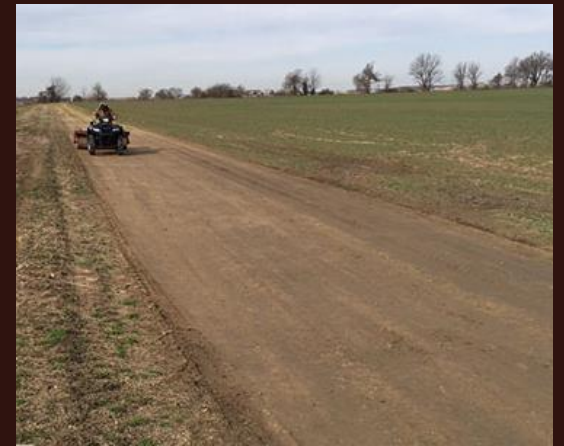
ROAD-HARD FINISHED ROAD
