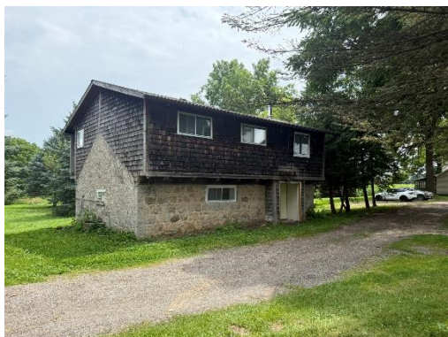
Milkhouse Exterior - Existing
