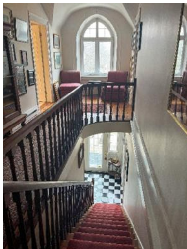
Stone House Second Floor Stair - Existing
