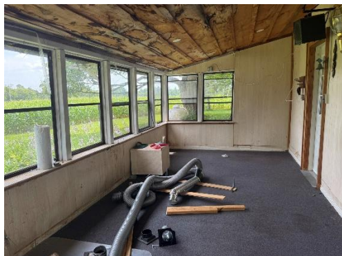
Duplex Screened Porch- Existing
