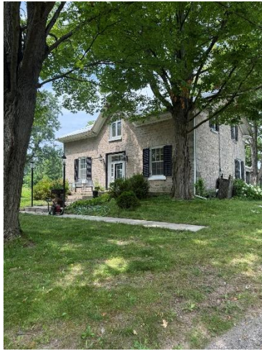
Stone House Front - Existing
