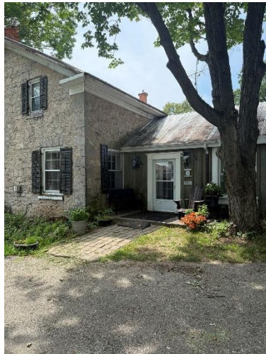
Stone House Side Entry - Existing
