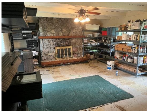
Duplex Living Room - Existing
