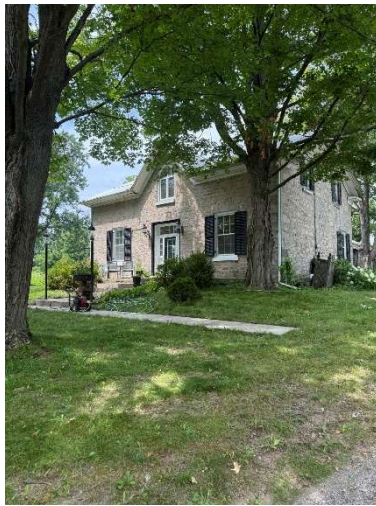
Stone House Front - Existing
