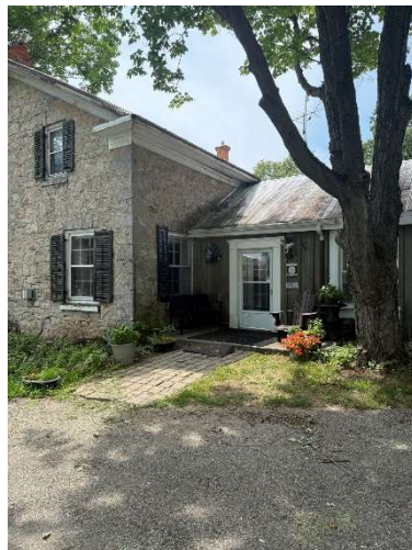
Stone House Side Entry - Existing
