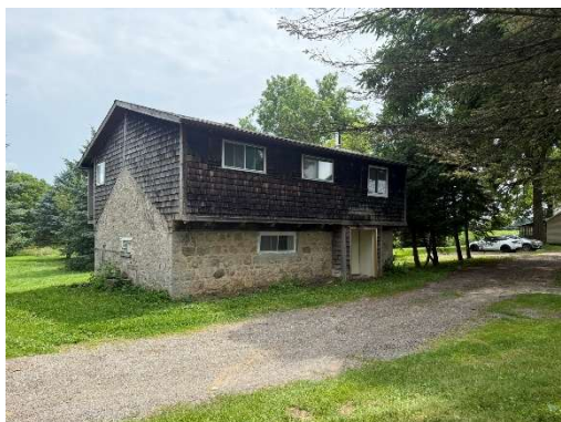
Milkhouse Exterior - Existing
