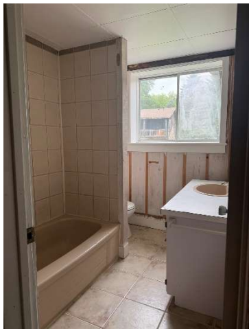
Barn Loft Bathroom - Existing
