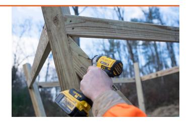
Measure from corner to corner as shown to make sure your leg structure is not twisted before finishing your angle brace attachment.
