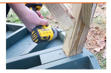
When all of the angle braces are installed they will create an X on each side of the tower stand as shown here.
