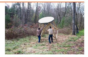
Place a level on the braces between each of the legs to determine if the stand needs to be leveled. Wooden shims, or rocks can be used to build up the low sides. Alternately you can use a shovel to dig away soil under the stand foot that needs to be lowered.
