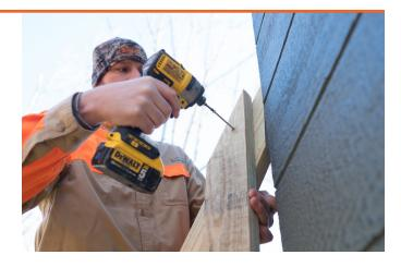
Fasten the railing to the stairway posts as shown.
